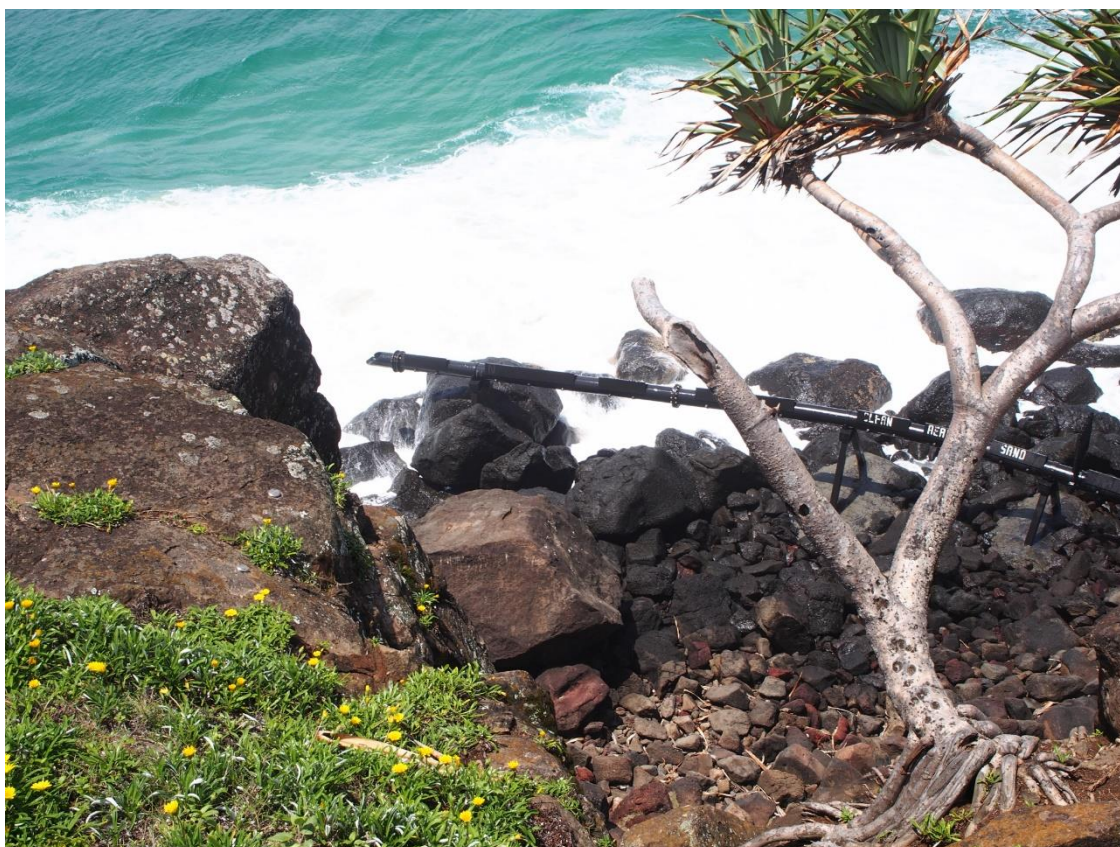
Figure 3.2 90% of the sediment bypassed through pumping is released at the coast of Snapper Rocks East. The pipeline is located above the water surface and releases the sand directly into the sea. Picture taken from the lookout point at Duranbah by DHI on 2017-11-08 shortly after high tide.
