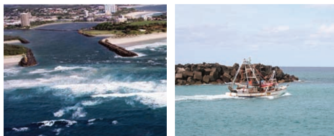
Hazardous navigation conditions at Tweed entrance in 1995, prior to sand bypassing (left), and Tweed River entrance today still requires caution.
